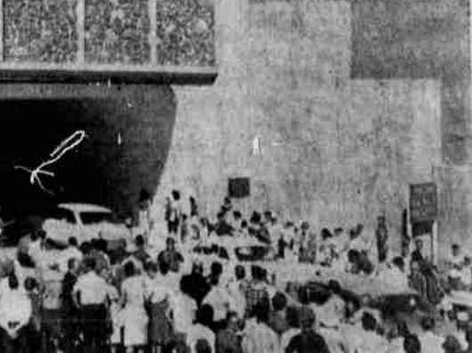
THROUGH THE TUNNEL — California State Sen. Randolph Collier's auto leads the procession of the first cars to go through the newly dedicated tunnel that is the finishing link on the Winnemucca-to-the-Sea Highway. Dignitaries from Oregon, California, Nevada and Arizona were present at the dedication rites. — UPI Telephoto
