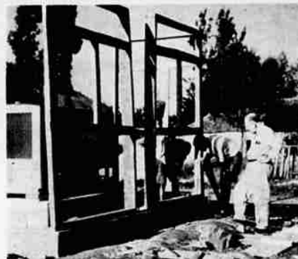
Dr. Lalonde oversees clinic construction.
