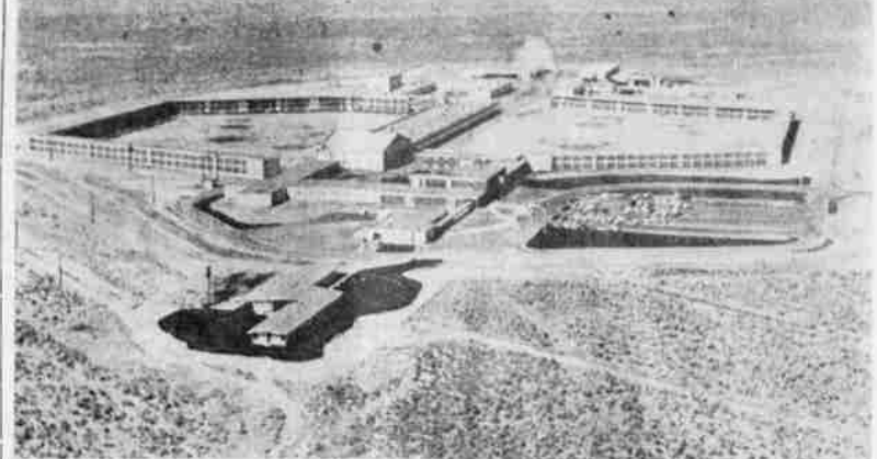
NEW CORRECTIONAL CENTER — This aerial view shows the nine million dollar correctional center that opened in Susanville, Calif., Saturday. The center, a pioneering concept in correctional programs, will hold 1,200 minimum and medium security state prisoners and is designed to save men by putting them to work saving the state's natural beauties. The center, first of four throughout California, will teach men how to fight fires, replant burned-over forests, combat forest insects, clear streams and perform other conservation tasks.
