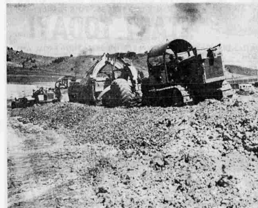
OTI WORK ADVANCES —Construction work on the shaping of the new campus for Oregon Tech, including work on the nuclear fission building and preparation for additional structures, is moving rapidly ahead as the $6,500,000 campus moves toward its deadline of the fall of 1964. Most recent construction bid awards call for an administration building, physical education building, physical plant building
