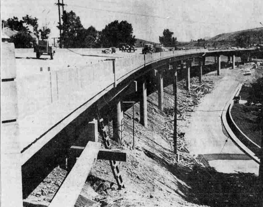
SPAN BEING PREPARED —This view, taken from the portion of the bypass just above Conger Avenue, looks out across Lake Ewauna and down the length of the new bridge span that crosses Main Street at this point. The completed project will cost an estimated $861,000 and is scheduled for completion by the end of 1963. Recently, the huge steel girders, 115 feet in length, were moved into place to cover the gap just over Main Street. Work will now move rapidly ahead on the completion of the bridge proper. Considerable work yet remains on the road structure on the south end where it is scheduled to link up with Riverside.
