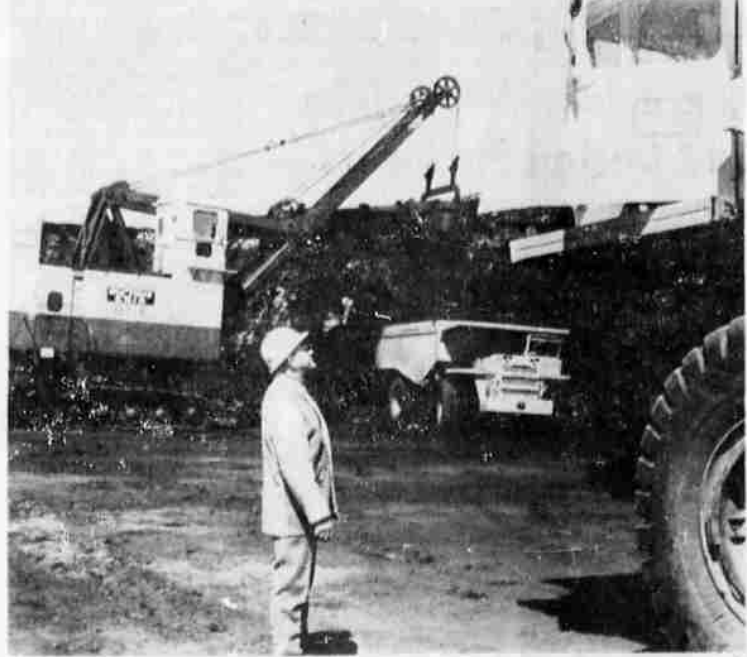
COAL FOR THE FURNACES — Almost 3,000 tons of coal daily pour through the boilers of the Dave Johnston steam generating plant just outside Glenrock, Wyo. In background can be seen one of the coal trucks being loaded. Each truck carries about 70 tons. The coal is conveyed through a long crusher assembly and reaches the burners in powder form. The coal comes from strip coal mines located south of the plant site and indications are that the supply will last at least 100 years.
