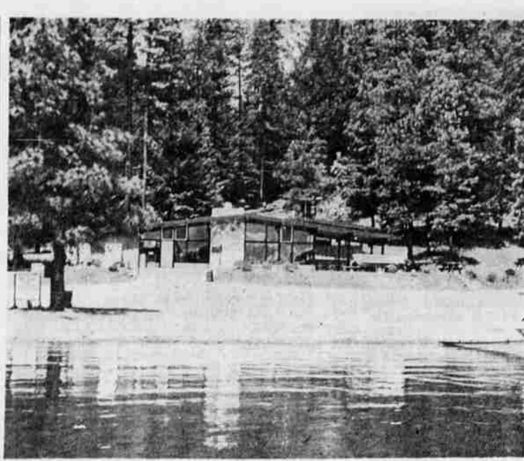
PARK'S CONCESSION BUILDING — This modern cafeteria and concession building at Howard Prairie Reservoir feeds many thousands of tired and hungry fishermen during the season from early spring to late fall. The "oasis" is an especially welcome sight around 10 or 11 a.m. on opening day when there's two feet of snow on the ground and the fish aren't biting. The store is equipped to provide many basic needs and accessories for weekend campers and fishermen.
