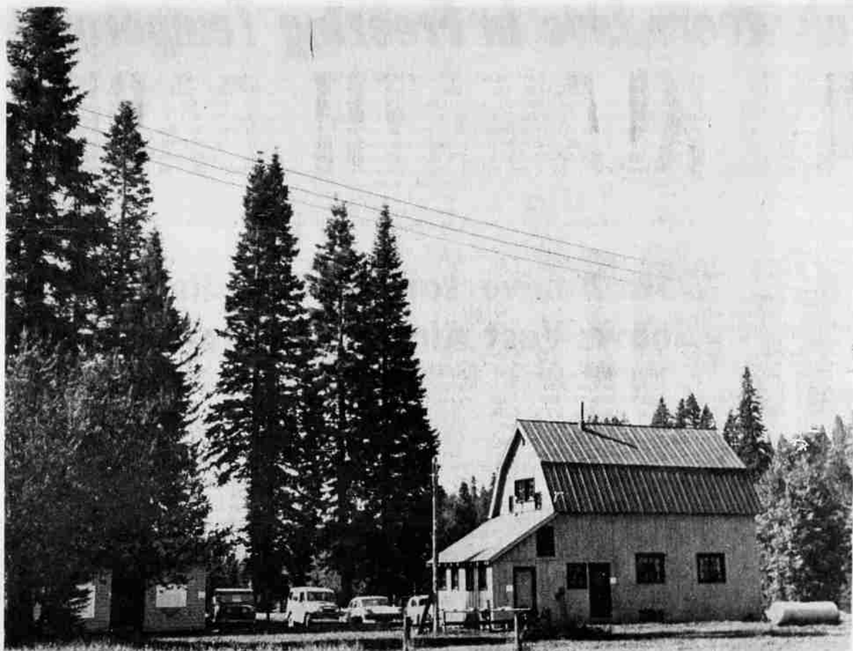
FIRE-FIGHTERS STUDY AMID TIMBER — A building used as a barn many years ago provides classrooms for fire-fighters of the Winema National Forest during the three-day fire school held annually in June at the Sevenmile Guard Station. This year 48 trainees took the instruc-
