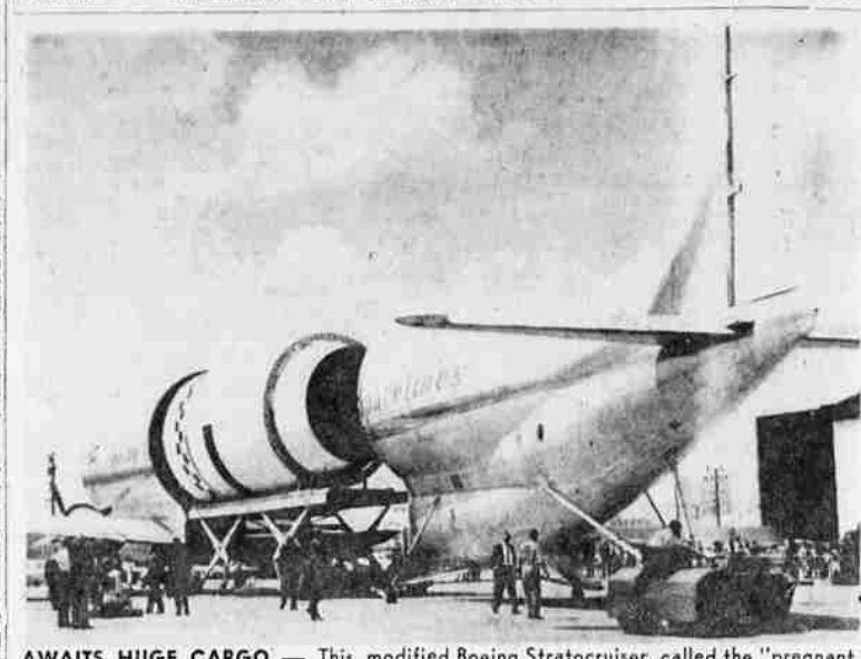
AWAITS HUGE CARGO — This modified Boeing Stratocruiser, called the "pregnant guppy," will carry part of the Saturn I space vehicle. The cargo weighs 20,379 pounds. This will be the largest cargo ever transported by airplane. The flight will be the beginning of loaded flight tests for the Federal Aviation Agency and the National Aeronautics and Space Administration.
