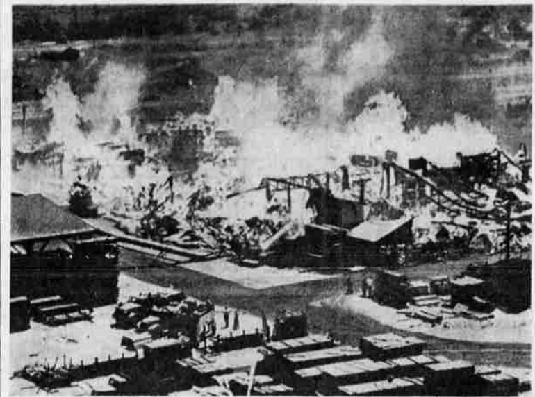
MILL FIRE AT EUREKA — This aerial photo shows wind-swept flames roaring uncontrolled through the planer mill of the Simonson Lumber Company on Highway 101 in Eureka Saturday afternoon. Stacks of over a million board feet of choice redwood lumber were also consumed. Firemen were unable to fight the blaze due to the intense heat from the flames.
