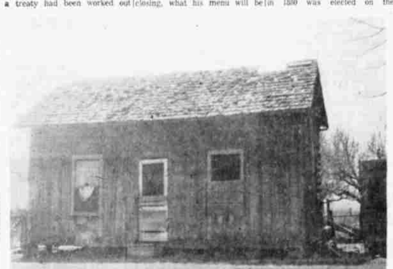
A LANDMARK — In 1936 this was the oldest house standing in Klamath County, built by O. A. Stearns in 1870 on land on the Keno Road which he bought from the state of Oregon. The frame house originally had four rooms with a porch across the front and was considered a fine home in pioneer days. The shingles on the house were made by hand by Oscar Stearns, a brother of O. A. Many prominent people were guests in this home and the owners always "kept travel." The original homestead joined this land. Members of the family still live nearby.
