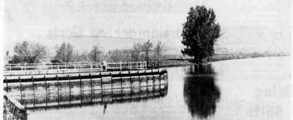
RESERVOIR SPILLWAY — A solitary angler appraises the spillway of the reservoir near Spring Creek Road before casting his line into the placid waters in the foreground. Other fishermen tested that part of the reservoir behind the spillway with varied success.
