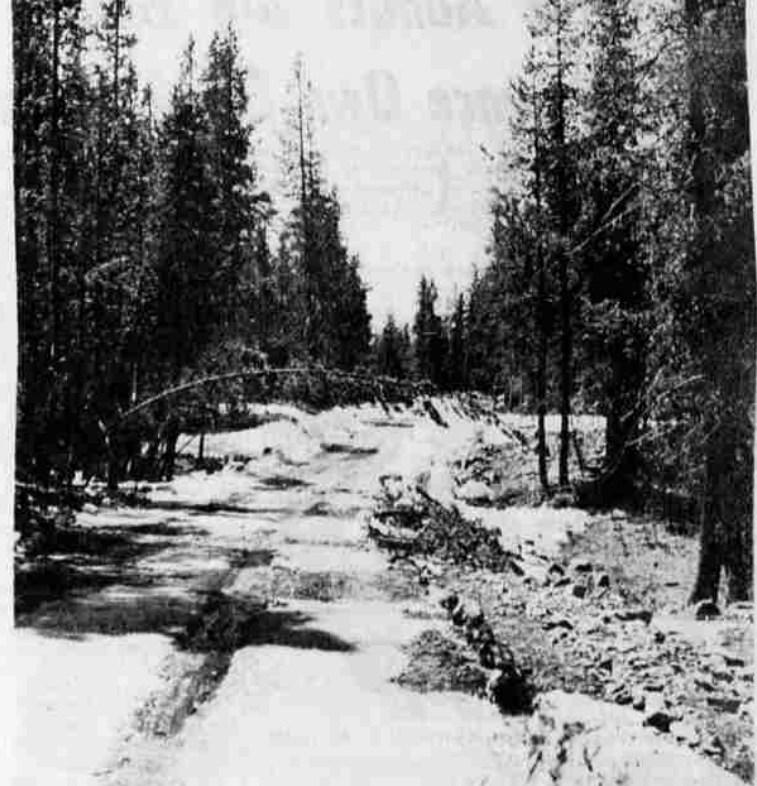
LOW BRIDGE AWAITS BOAT CARRYING AUTOS — Slushy roads bordered with snow awaited anglers venturing into Four Mile Lake and Fish Lake during the opening of the fishing season in the high mountain country west of Klamath Falls last Sunday. In photo above, a partially fallen evergreen, extending across Four Mile Lake road, complicated the problems of those anglers who carried boats on the tops of their cars. Fishermen equipped with car-top boats stopped their vehicles in front of the tree and motored slowly under it. Fishing was generally slow in the two lakes during the opening day weekend.
