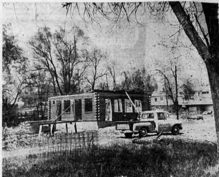
DRIVE-IN GOING UP — A new drive-in, to be called "Tio-Toms" is being constructed on Biehn Street and plans call for it to be operating early in June. Eric Lewis and Gail Sigmund are partners in the new venture which will feature complete drive-in service and a 12-stool counter. The partners are contracting the building and estimate the cost at about $12,000 for the structure. It is made of Redi-Cut logs.
