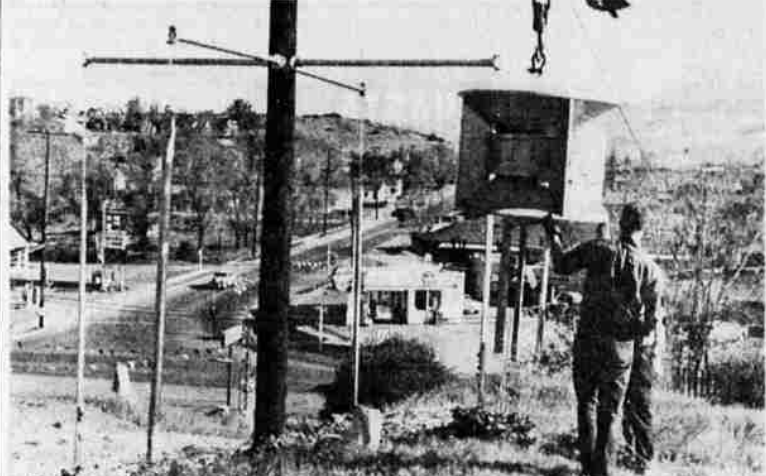
FIRST SIREN BERTHED ON POWER POLE — The first air raid warning siren ever installed in Klamath Falls was unceremoniously hoisted up and affixed to a power pole at Lakeview Avenue and Trinity Street about 8:30 a.m. Thursday, by three employees of the Roseburg Fire Equipment Company. Three other sirens were also to be erected elsewhere in the city this week, and will be supplemented later in the year by three more alarms, which will complete the seven-siren system. The Roseburg firm entered the low bid of $6,485.75 for the sirens, including installation. Story, Page 4A.
