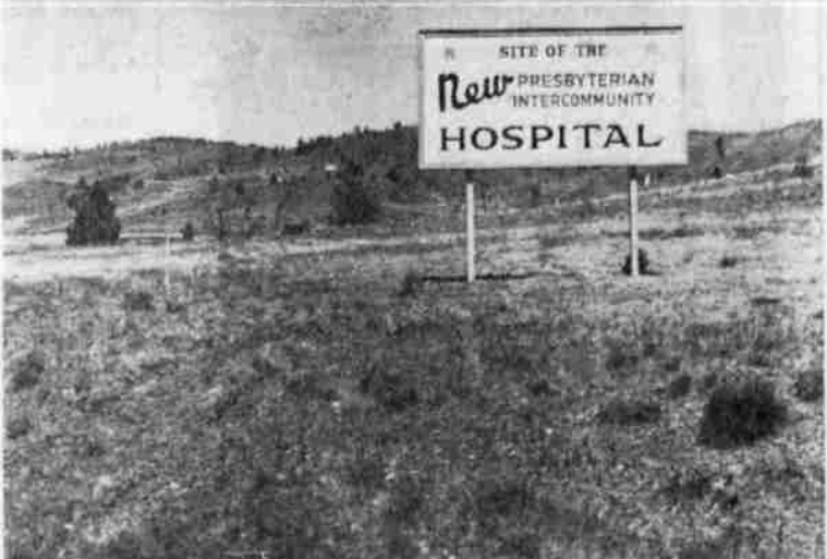
HOSPITAL SITE DEDICATION — The first formal step toward construction of the new Intercommunity Hospital is set for 2:45 p.m. Sunday, in the form of the dedication of the hospital site, located adjacent to the new OTI campus in McLoughlin Heights. Sen. Barry Goldwater of Arizona will be guest speaker at the site, which is to be dedicated by Rev. John O. Reynolds of the Medford Westminster Presbyterian Church. One-third of the three million-dollar project has been contributed by residents of the Klamath Basin with most of the remaining funds to be obtained from the Accelerated Public Works Program or Hill-Burton Funds. To reach the site, go north of Klamath Falls on Highway 97 and turn right onto the new OTI campus access road. Drive to the end of the road where attendants will guide motorists to parking facilities.
