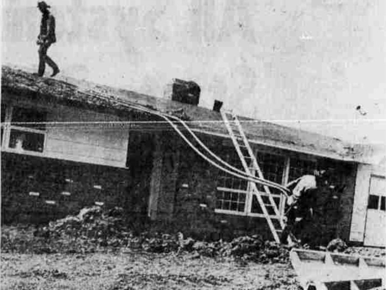
ROOF BLAZE EXTINGUISHED — City firemen prepare to return to the fire station after putting out a tarpaper blaze on the roof of a home under construction on Calhoun Street. Firemen arrived at about 1:50 p.m. Tuesday before any serious damage was done to the roof itself. A tar mop left to dry on the roof was whipped aflame by a breeze setting ablaze the freshly laid tar on the roof. The $30,000 home is owned by John Tyrholm. The Tyrholms were preparing to move into the home in about two weeks.
