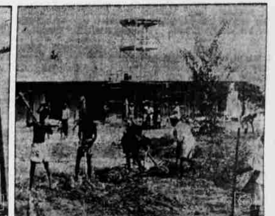
Native crew puts finishing touches on Project Mercury telemetry building at Kano, Nigeria, one of a world-wide network.
