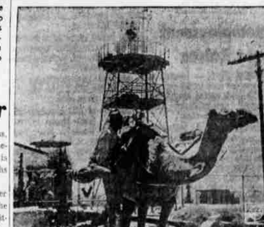
Local transportation was pressed into service—in this case, a camel—during station construction on Grand Canary Island.
