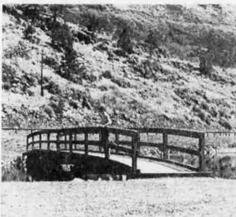
BRIDGE ACROSS BARCLAY SPRINGS
