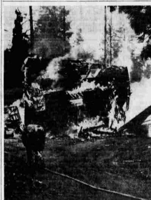
NOTHING LEFT —Here, a fireman begins to roll up the hose as the last wall of the Esperen home tumbles inward in the background. Firemen could only keep the surrounding trees and shrubbery wet down so that the flames would not spread. When they responded to the 9:01 a.m. alarm flames had already virtually completely enveloped the home on Lakeshore Drive.
