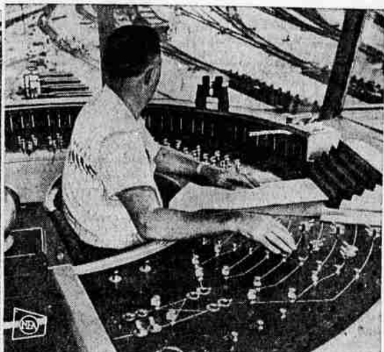
AUTOMATED CONTROL — This is a view of the interior of an automated freight yard control tower panel. Few railroads have these efficient electronic systems.
