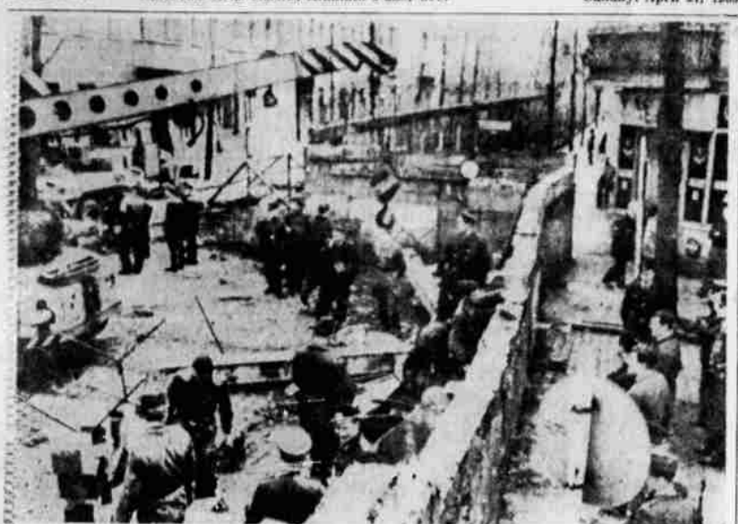
WALL REPAIRED AFTER CRASH — East Berlin policemen on the left side, repair the Berlin Wall Thursday as West Berlin police and others gather on the right side. This is the section of the wall that was damaged Wednesday when Wolfgang Engels, 19, a mechanic, rammed a Communist armored car into the structure while escaping into West Berlin. Shot during the escape, he was recovering from an emergency operation in West Berlin. — UPI Telephoto
