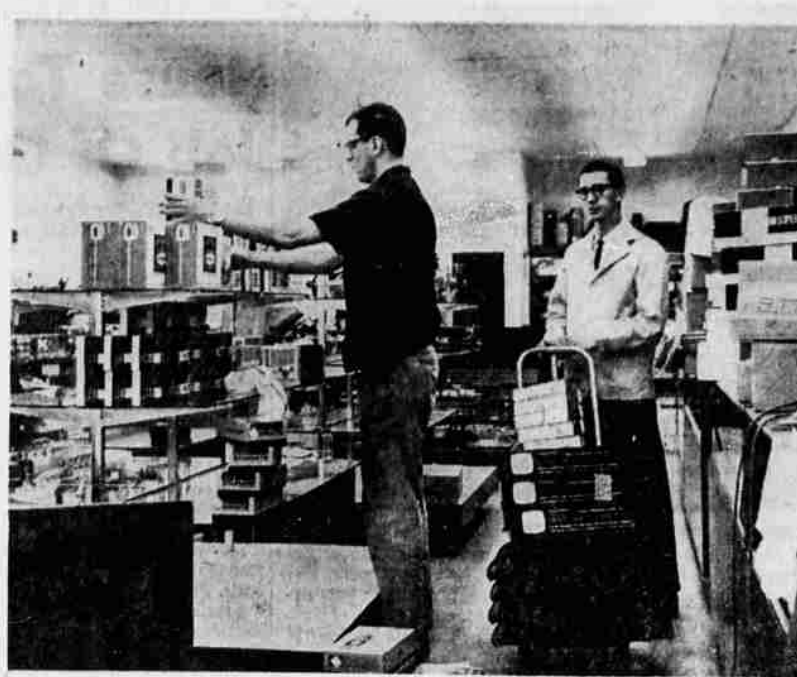
FINAL TOUCHES — George DeShiell, left, and Bob Gates, are busy with last minute touches of displays at the new quarters of Weisfield's, corner of Seventh and Main. The firm offered special grand opening bargains throughout the store beginning today. Norman Burns, manager, indicated that the bargains and the grand opening will continue through Saturday. The new location, across the street from the old, has been completely remodeled, inside and out. A complete list of grand opening bargains was included in a special section of the Wednesday Herald and News.
