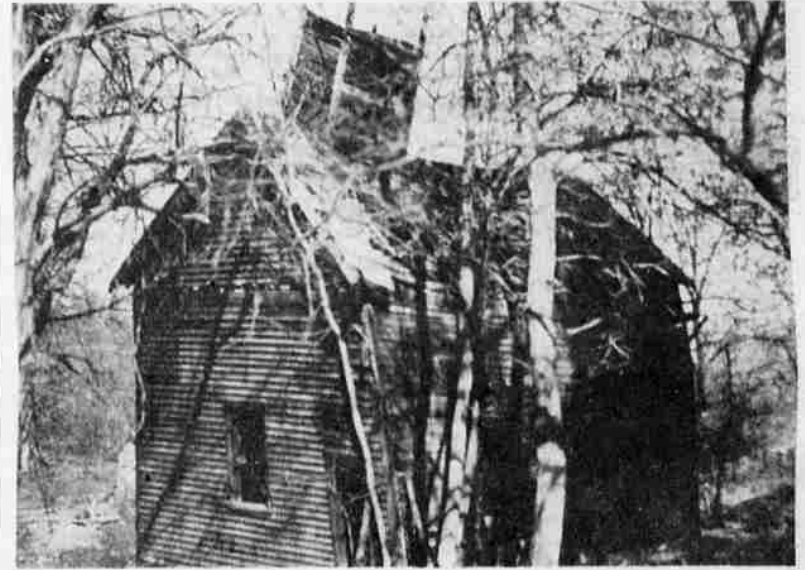
OLD DEHYDRATOR — The Forest House orchards were once both productive and profitable, so a fruit drying house was built in 1860 to dry the apples, pears, peaches, and plums for the packing and canning operations which were established on the ranch. It served its purpose for many years, but it was in such a decrepit state that it was necessary to tear it down several weeks ago.
