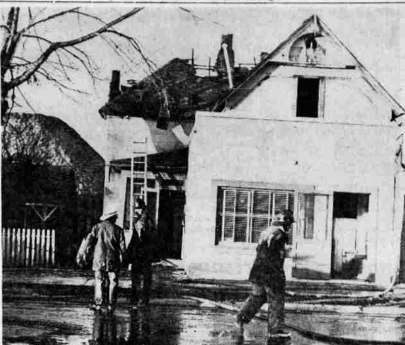
FIRE GUTS ROOMING HOUSE — Klamath Falls firemen stand outside a rooming house that was gutted by fire which started sometime before 3:30 a.m. Sunday. The building was owned by Mrs. Leona Boyles, who discovered the fire when she returned from a dance. Two elderly roomers who were sleeping upstairs got out of the building safely. One of the men was found near collapse on the staircase by a fireman. Fire Chief Geno Gheller said it was the worst house fire in the city in years.
