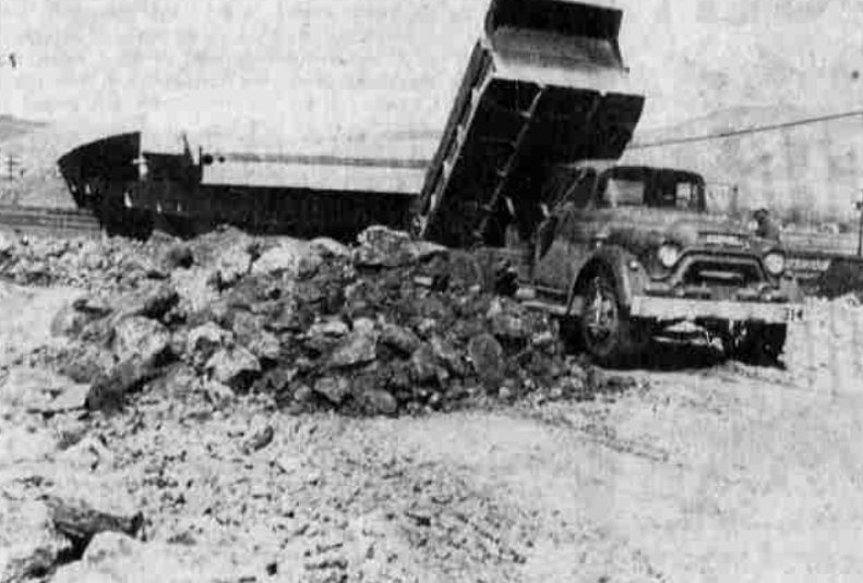
constructed by the Inter-City Construction Company of Eugene at a cost of $29,504 and is scheduled for completion about the end of April. As workmen of the Eugene construction firm were driving pilings into place to support the Alameda Avenue bridge, employees of the county road department were laying dirt fill (photo at right) to build the second of two approaches to the overpass near Laverne Avenue at the southern end of Washburn Way. The approach work, slated for
