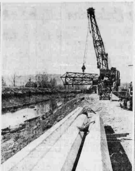
BRIDGE GOING UP — Construction workers today began driving concrete pilings which will support a bridge that will carry vehicular traffic proceeding between Washburn Way and Alameda Avenue. Work on the new bridge, being constructed by the Inter-City Construction Co. of Eugene at a cost of $29,504, was started last Wednesday when the firm began hauling in materials for the job. Above, workmen begin moving a part of the crane into place before fitting it to the crane housing. The crane is in operation on Washburn Way, across from Alameda Avenue, located on the other side of the canal.
