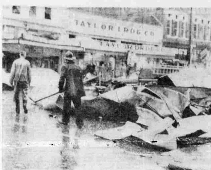
TORNADO DEBRIS — Firemen work Wednesday in Bessemer, Ala., to clear the streets of roofing, signs, and other debris from a tornado that ripped into a two-block section of the downtown business district. — UPI Telephoto
