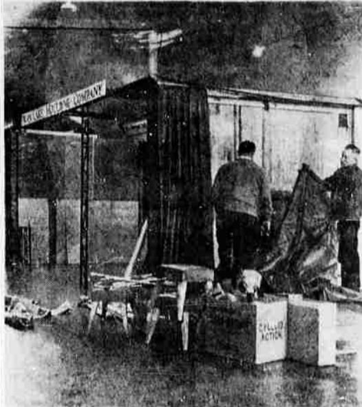
GETTING READY — Here, two persons are getting ready one of the displays that will be shown at the Home Show at the Klamath County Fairgrounds. Booths were built by members of the sponsoring Kiwanis Club, and each exhibitor arranged his own display.
