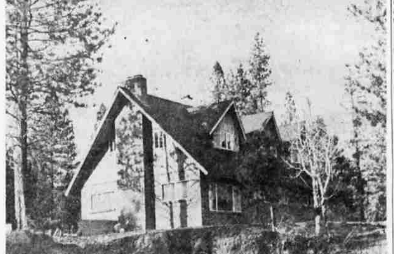
NEW HOME — Mr. and Mrs. Peter Macfarlane and their seven children moved into this six bedroom two-story home on a bluff just west of U.S. 97, adjacent to the Chiloquin junction and the family service station business. Landscaping is planned for the future. The home is one of several new ones which were completed in the area last year.
