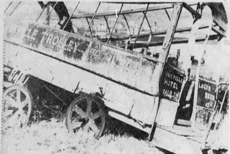
ABANDONED — This was the ignoble end for the once proud Sutter Street trolley which once graced the streets of early-day Klamath Falls. Abandoned, it fell victim to fire, and then gradually disintegrated into junk. Today a few pieces still lie in some secluded corner at Moore Park, all that remains of the only streetcar that ever graced the streets of Klamath Falls.
