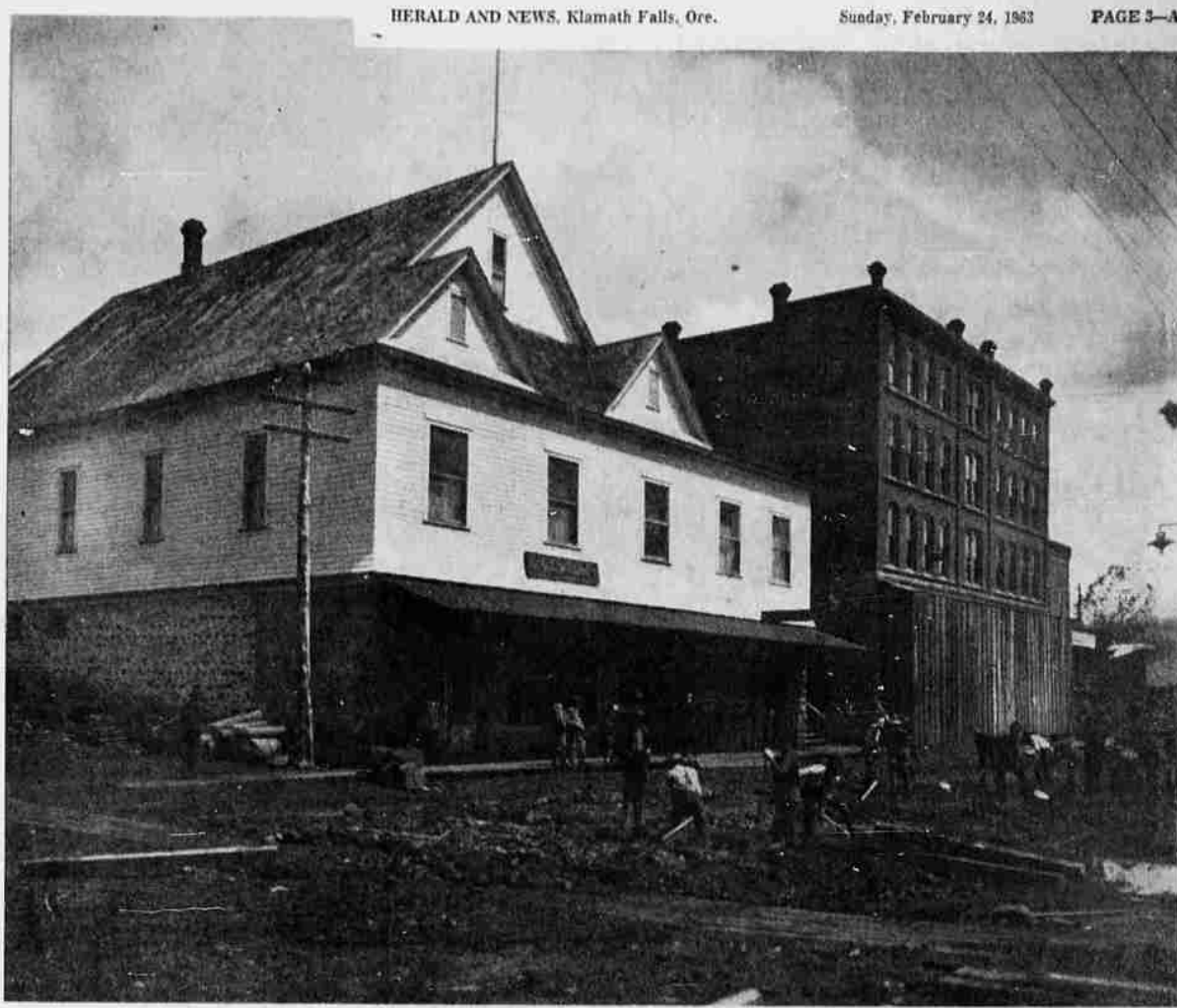
Note that the front of the Baldwin Hardware Store (now Baldwin Hotel) has been boarded up. It was understood that dynamite had to be used in some spots to loosen the rock, although this fact has not been confirmed. In view at right, photographer on this day in 1906 moved up closer for a view taken from the wooden sidewalks which
