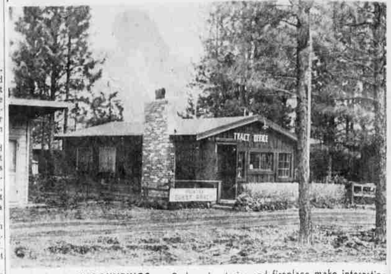
ATTRACTIVE SURROUNDINGS — Redwood exterior and fireplace make interesting spot for signing on the dotted line for a lot at Frontier Guest Ranch. Family living quarters for the Harold J. Fish family are in rear.
