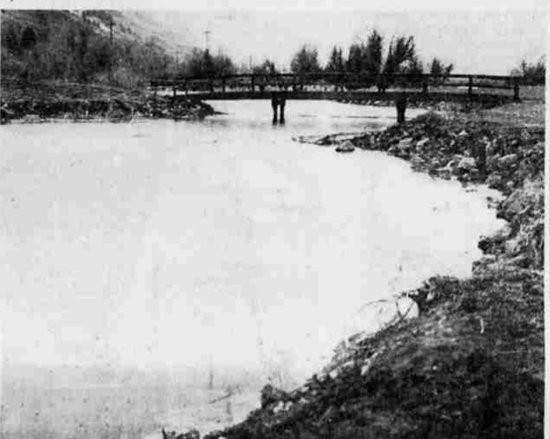
LANDSCAPING NEXT PROJECT — Rain muddies the usually clear stream, intersecting Hagelstein Park, which has been partially completed at a cost to the county of almost $19,000. The banks of the stream and land elsewhere in the park will be landscaped beginning this year. Construction of the bridge and fencing of the area has been completed as part of the program to construct the park.
