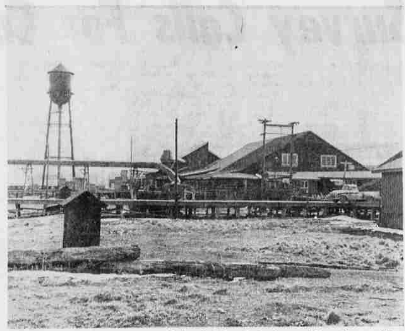
OLD PLANT — This is one view of the old Klamath Lumber and Box plant in Shippington Addition which went under the auctioneer's hammer in March of 1962.
