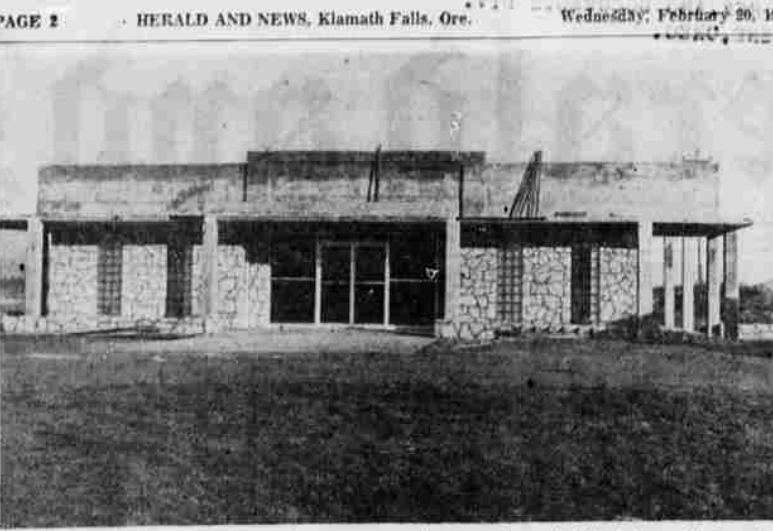
NEARING COMPLETION — The new mausoleum at Eternal Hills Memorial Gardens is expected to be finished by Memorial Day. The structure awaits arrival of marble from Italy and Portugal. All concrete work, the office, flower room and rest rooms are completed. Mr. and Mrs. Edward J. White, owners, will also place a lighted stained glass window in the end of the building and will landscape the grounds. The cemetery, newest in Klamath Falls, is located on the Merrill Highway.
