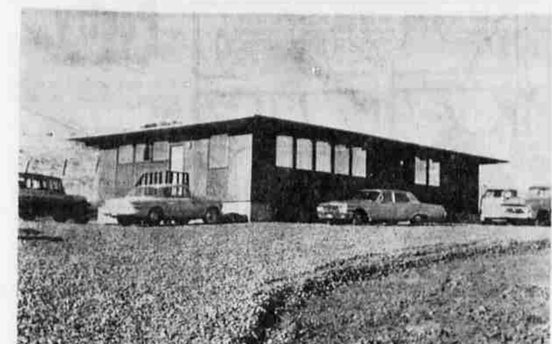
NEW OFFICE BUILDING — Klamath Lumber and Box Company has moved into its new office quarters which was just completed by Warren Parr, contractor. The building is 32 by 56 feet made of post and beam construction and was started in late August. It has a half basement. Estimated cost of construction was in excess of $30,000.
