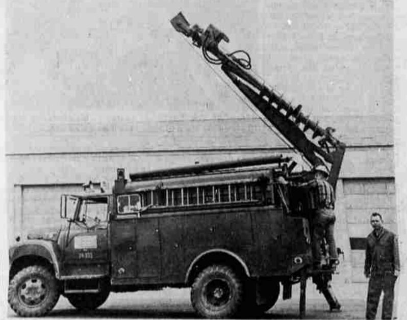
NEW AUTOMOTIVE EQUIPMENT — The newest rig obtainable is brought out for inspection. Costing $20,000, the new rig provides a powered digging arc of 180 degrees with the power takeoff at the rear. Here, equipment operator Glenn Clevon prepares to demonstrate the equipment while Roy Rolfs, superintendent of the service center, looks on.
