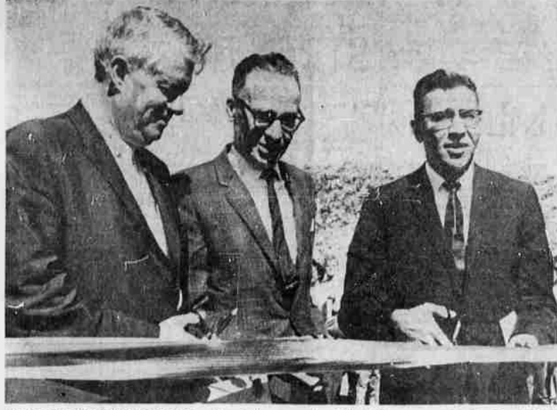
IMPORTANT ROUTE OPENED —The last segment of the Winnemucca-to-the-Sea Highway was dedicated on Saturday, Sept. 22, with a special ribbon cutting ceremony at Doherty Slide about 70 miles east of Lakeview. In this photo representatives of three states participate in the ribbon cutting. Left to right, Sen. Randolph Collier, California; Sen. Harry Boivin, Klamath Falls, and Gov. Grant Sawyer of Nevada. J. Vern Owens, Klamath Falls, was emcee for the program.
