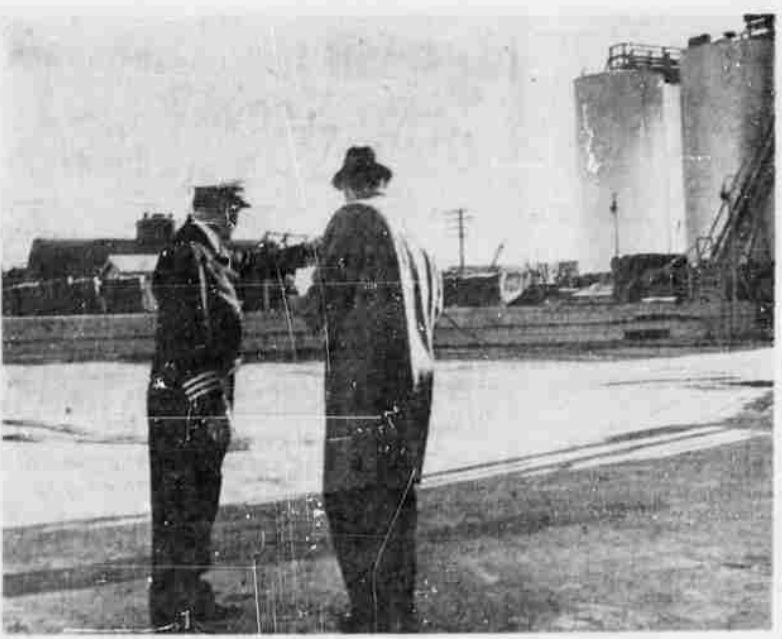
DANGEROUS GASOLINE LEAK - Fire Chief Geno Gheller shows Herald and News reporter George Alotrico the gasoline storage tank at the Shell Oil Company bulk plant on Spring Street that lost about 20,000 gallons Wednesday morning.
