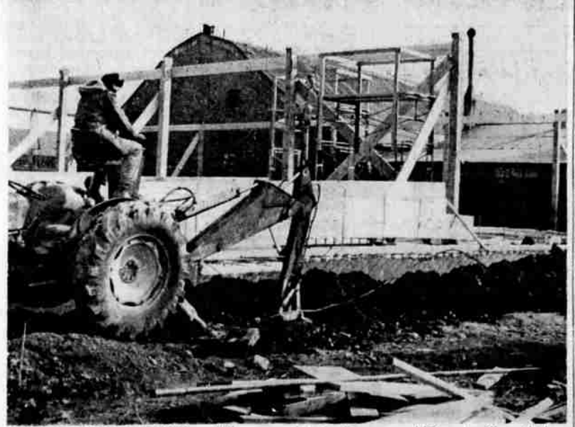
NEW STORAGE ADDITION — When completed, this new addition to Klamath Ice and Storage Company on Spring Street will give the company room for another five million pounds of storage. It will be used for frozen food storage and also for local potato storage. It is expected to be ready for use by the first of the year.
