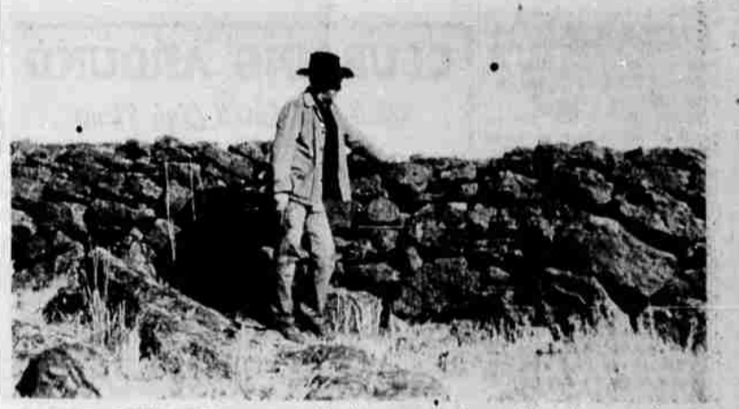
IF STONES COULD TALK — Probably few persons live today who remember the building of the stone wall on the Jesse D. Carr Ranch near Clear Lake. But the stories of the building of that wall are legion, some fact, some legend. The wall "shoulder high to a horse" kept cattle herds inside on Carr land and near water, but it also kept out other livestock and land seekers, according to all newspaper records. Devere Helfrich stands beside part of wall still intact on north side of Clear Lake near old ranch headquarters. The wall was built between 1875 and 1882.
