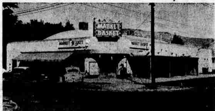
MARKET BASKET at South 6th and Shasta Way — a completely remodeled super market — and we're holding the Grand Opening this weekend!
