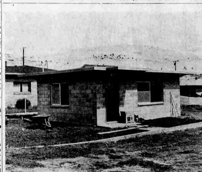
NEW QUARTERS — This pink pumice tile building on Hilyard Avenue is headquarters for the Enterprise Irrigation District. The building accommodates the office where Gerald West is office manager. George D. Kohler, Hager, is district manager. Board members for the district are Dean Mercum, who built the structure, Bill Cunningham, Joe Keller Jr., Raymond Batty, and Everett Dennis. The district serves more than 2,000 water users.
