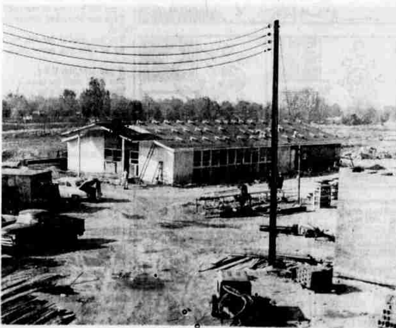
SCHEDULED FOR DECEMBER COMPLETION — The city schools' administration garage-warehouse unit nears completion at the Ponderosa School site. School officials expect to occupy the offices by December. The garage-warehouse section is seen (brick wall) going up at right; offices are located in the central building.
