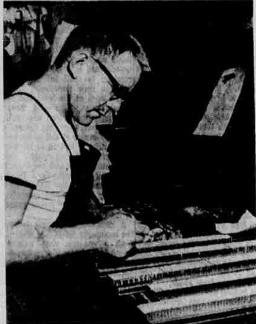
MAKING UP — Here, Charlie Zumwalt, makeup editor, is busy at work selecting the type that will be used to make up the day's newspaper. Hanging before him is a sample sheet, called a "dummy," which shows where the news editor wants various stories placed. The time-consuming task of cutting and fitting a story to its appointed place is done skillfully and quickly by Zumwalt and others in the makeup department.
