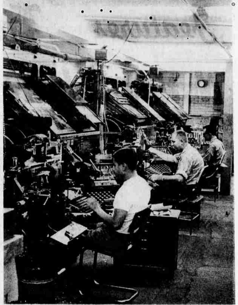
LINOTYPE OPERATORS — Punching out the daily copy for the newspaper is the task of these men in the composing room. Left to right, seated at linotype machines, are Nick Valdez, Lorne Allen and Jerry Morgan. It is specially adapted machines of this type which are operated by the perforated tape on the same principle as the old player pianos.
