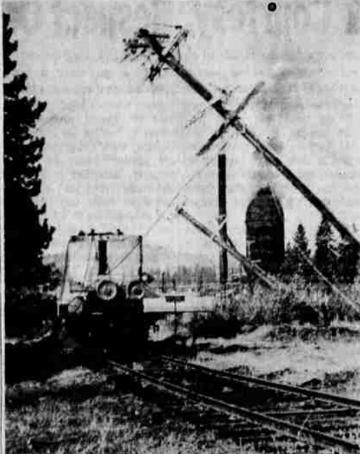
RIPS OUT POWER — This McCloud River Railroad car, carrying a log-loading crane, ripped out power, telephone, fire alarm and signal wires Friday in McCloud; crippling communications in that city. Brake failure was blamed for the accident. Two cars rolled down an incline, struck a derail switch and left the track. The crane's boom swung wildly through the air and ripped down the lines. One power pole was broken and four left standing at 45 degree angles.
