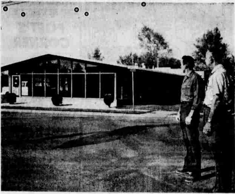
NEW OFFICES — The Pacific Gas Transmission Company has moved into these office quarters at the corner of East Main and Wantland. Guy W. Goodman, district foreman for this district for the firm, indicated that the maintenance crew for the natural gas pipeline will operate out of here for this district which runs from Crescent to the California-Oregon state line. The staff consists of three men now, and will be 11 men when fully staffed. Goodman is shown here at right, with Vance Crouch, clerk and warehouseman.
