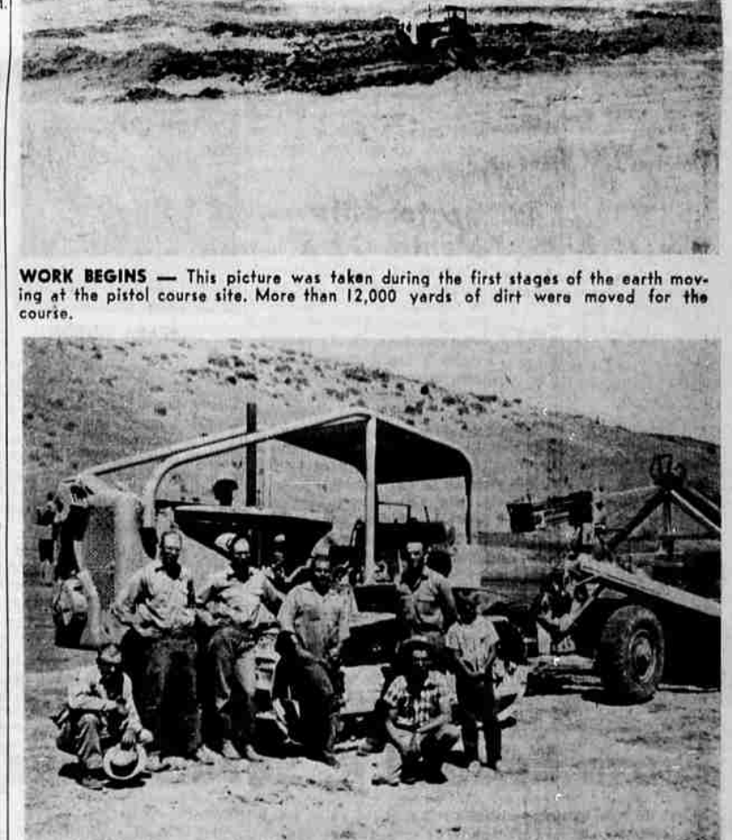
CAT WORK — Operation of the heavy machinery at the pistol range site was handled by these men. Left to right, standing, Dale Ellis, Chuck Ellis, Phil Chlopek and Archie Huff. Kneeling, left, Amos Kelsey, Sgt. John Kennard, and Kennard's son David. The operation required more than 155 hours of heavy equipment.
