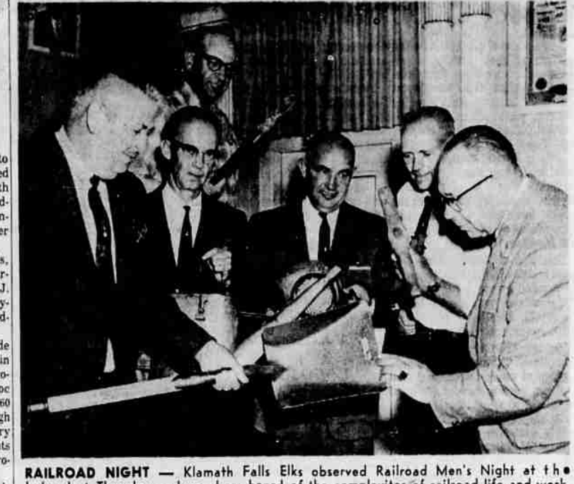
RAILROAD NIGHT — Klamath Falls Elks observed Railroad Men's Night at the lodge last Thursday and members heard of the complexities of railroad life and work. Showing Exalted Ruler C. M. Gilmore some of the tools of their trade are, left to right, Homer Bissell, Marion Foster, Gerald Rutledge, Sam Burton, Dick Hayden and Gilmore.
