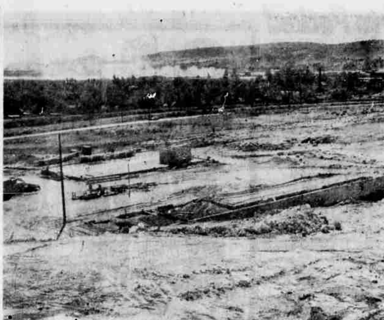
WALLS BEGIN GOING UP — The new Klamath Falls city schools administration unit, garage and repair facility near Ponderosa School. Construction will be finished, the contractor estimates, by Dec. 1; school officials estimate moving into the new structure will take place during Christmas vacation.
