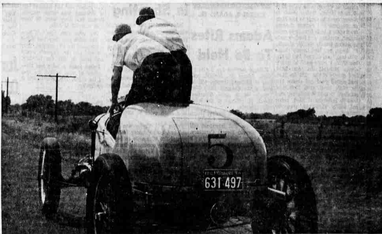
Shell Research scientists, Dave Berry and Fred Schuette, in the rebuilt 1924 coupé which set the world mileage record. Its original frontal area was reduced by about 75 per cent to cut down wind resistance. Shellzone® anti-freeze was
